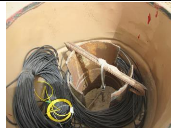
Figure 1. Wellhead of smart DAS uphole before installing protection cover.
