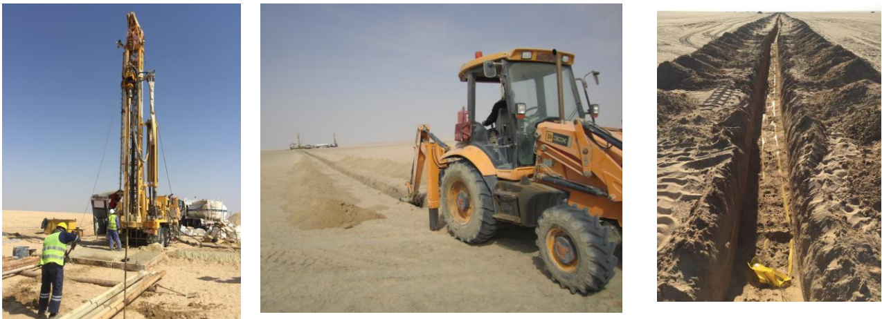
Fig. 8—DAS Uphole drilling and trenching.
