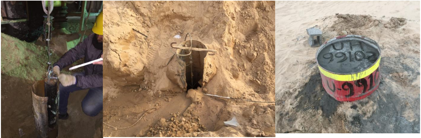
Fig. 9—DAS fiber installation and completion.
