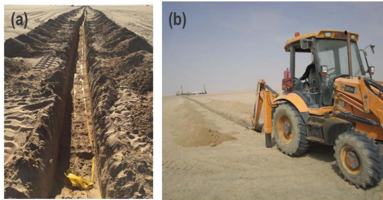
Figure 8—Horizontal trenching of a DAS cable at the surface.
