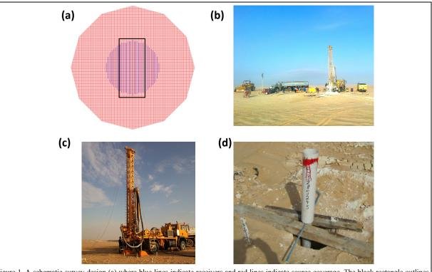
Figure 1. A schematic survey design (a) where blue lines indicate receivers and red lines indicate source coverage. The black rectangle outlines the area of interest. The drilling layout at one of the locations (b) and a portable drilling machine (c) along with a drilled location (d) ready for sensor installation.
